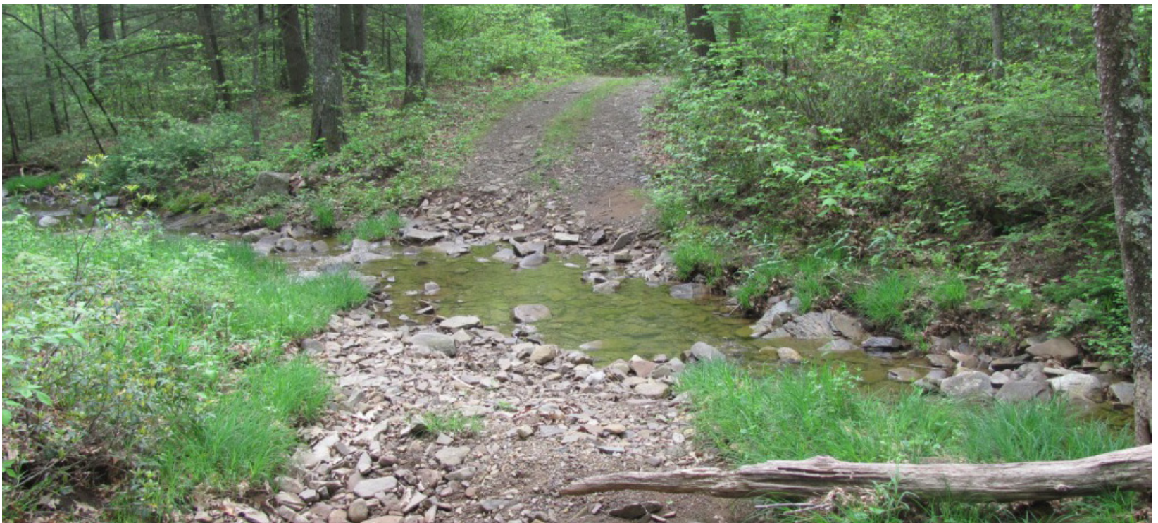
A stream crossing on Little Skidmore Road, where natural drainage is reasserting itself.
