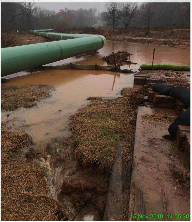
EXHIBIT G – The upstream side of the bridge over Little Creek. Muddy water flows under the bridge and out the downstream side of the bridge before entering the creek, seen in Exhibit H.
