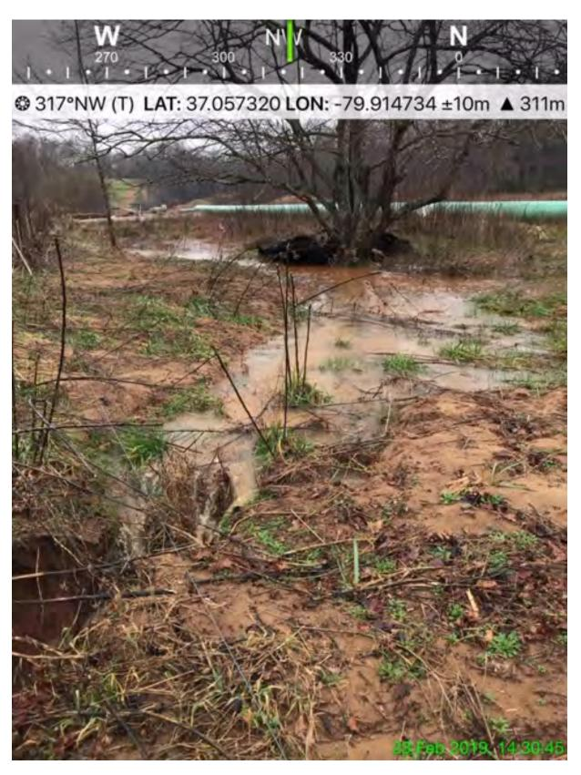
Exhibit E – Same location as in Exhibit D, two days later, after 2.5 inches of rain. The drainage into the creek is collapsing. The fence wire is visible on the left.
