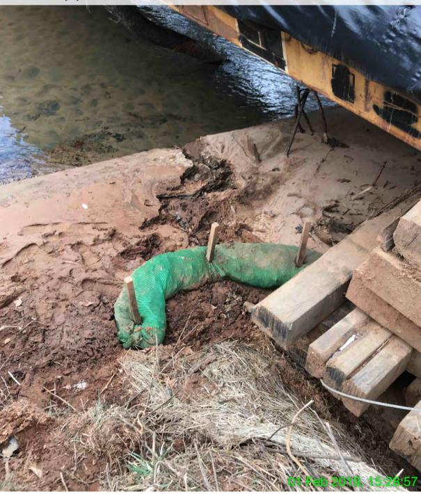
EXHIBIT I – The downstream side of the bridge over Little Creek which is the same location as Exhibit H above. The creek bottom which used to be rocky is covered in sediment. Sediment is piled on the banks. The erosion control sock had been recently installed when this photo was taken on February 1, 2019.
